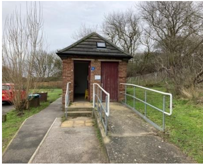
View of access to Gents and Disabled toilets
